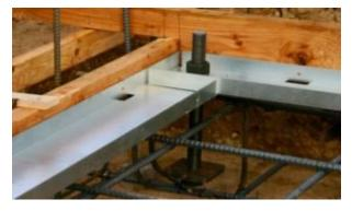
The nut holds the anchor bolt in place. The bolt must be tied off to rebar to ensure it is stable and plumb and will not move during the pour. This is the responsibility of the concrete contractor in cooperation with the general contractor.
