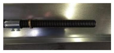
Electrical EMT connector acts as a stop under the template. Brass bushing fills oversized hole in template around anchor bolt. Step 5: Template Placement
