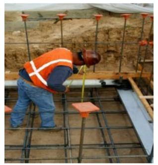
The bottom of the template is the top of the pit slab. Pit must be exactly 4 ft. deep with a level floor!!!!!
