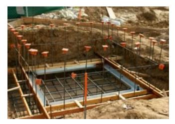
Template is now centered in the pit. Note colors in template at the corners, corner colors will match. Template is now ready to have concrete poured.
