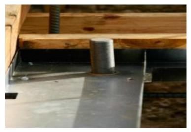
Anchor Bolt set in template. Notice brass ring, set before setting of nut. Note: a minimum of 9 ½ " of thread should be showing above template.
