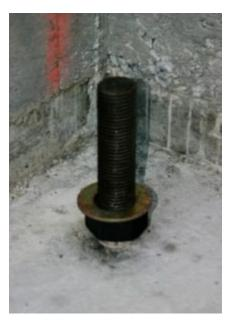
Completion of pit and view of bolt, ready to accept installation of elevator.
